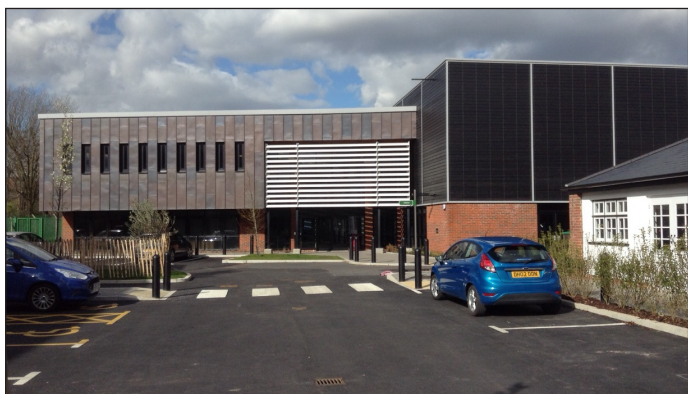
New Vale Lane Primary School
